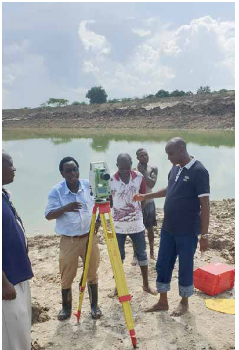
Taking Water Pan Levels at Nagele.
