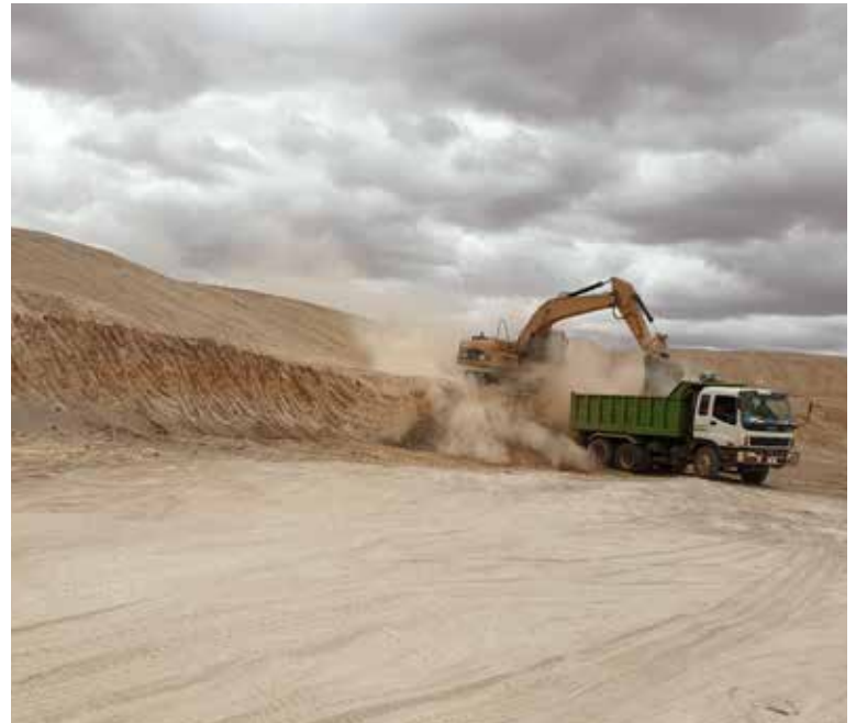
Water Pan Excavation at Boa in Wajir County
